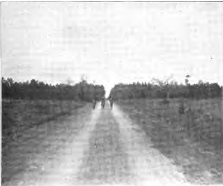
New Gretna road, Burlington Co., after improvement.
